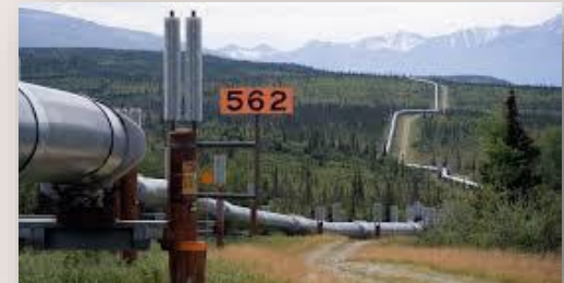
Single pipeline connection
